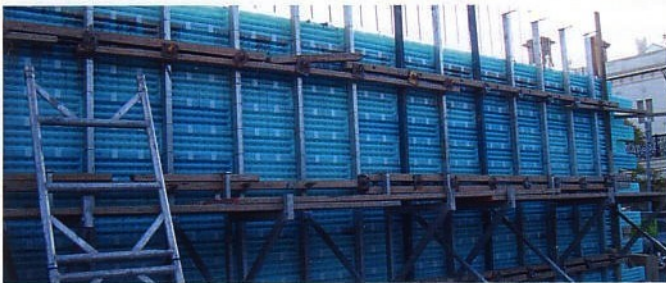
ICF plastic formwork in use on another recent Melbourne project.
