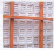
walls, they were not an option for the three upper levels because there was no crane access to the bottom of the 45 metre long by 12 metre wide site. "The project was originally designed for concrete blockwork, but when we had a look at the ICF Contracting system we were impressed with its versatility and cleverness," Grant said. "It's a much simpler and faster alternative than the old way of forming up with plywood."
